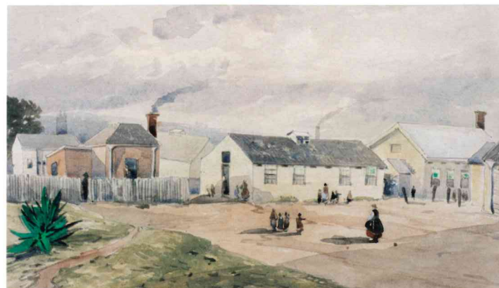
CAT NO 59 Industrial School, Geelong
