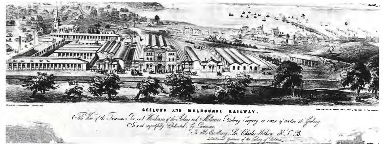
37. Edward Snell Geelong and Melbourne Railway. View of the terminus pier and warehouses of the Geelong and Melbourne Railway Company in course of erection at Geelong, 1854
